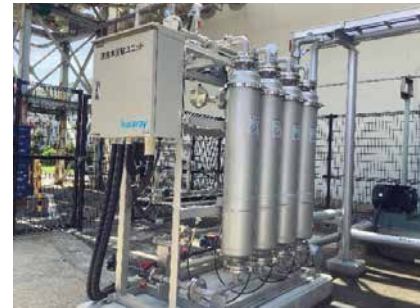
Membrane filtration facility
