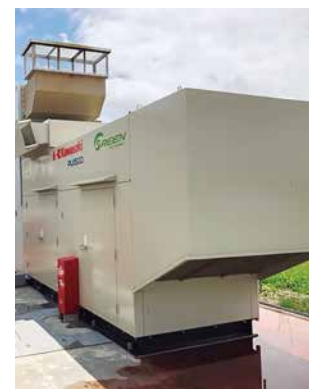
Emergency power generator (Taiki Plant)
