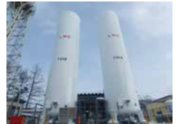
Liquid natural gas storage tank (Isobunnai Plant)
