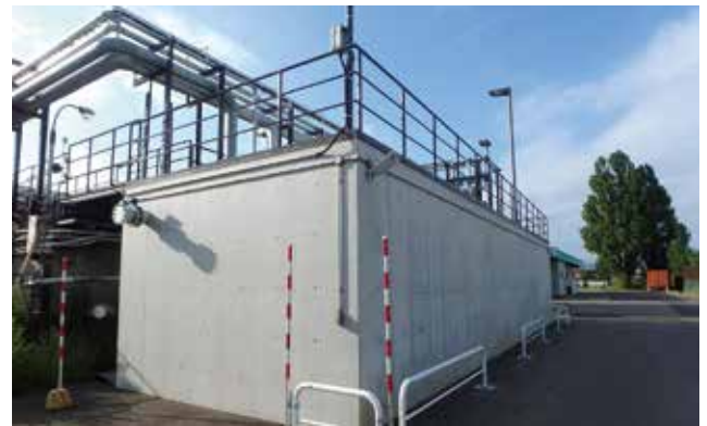
Wastewater treatment facilities (Sapporo Plant)
