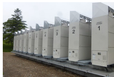
New energy-saving freezers installed on fresh milk intake facility (cooler station)
