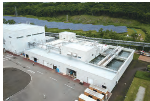
Wastewater treatment facilities (Isobunnai Plant)
